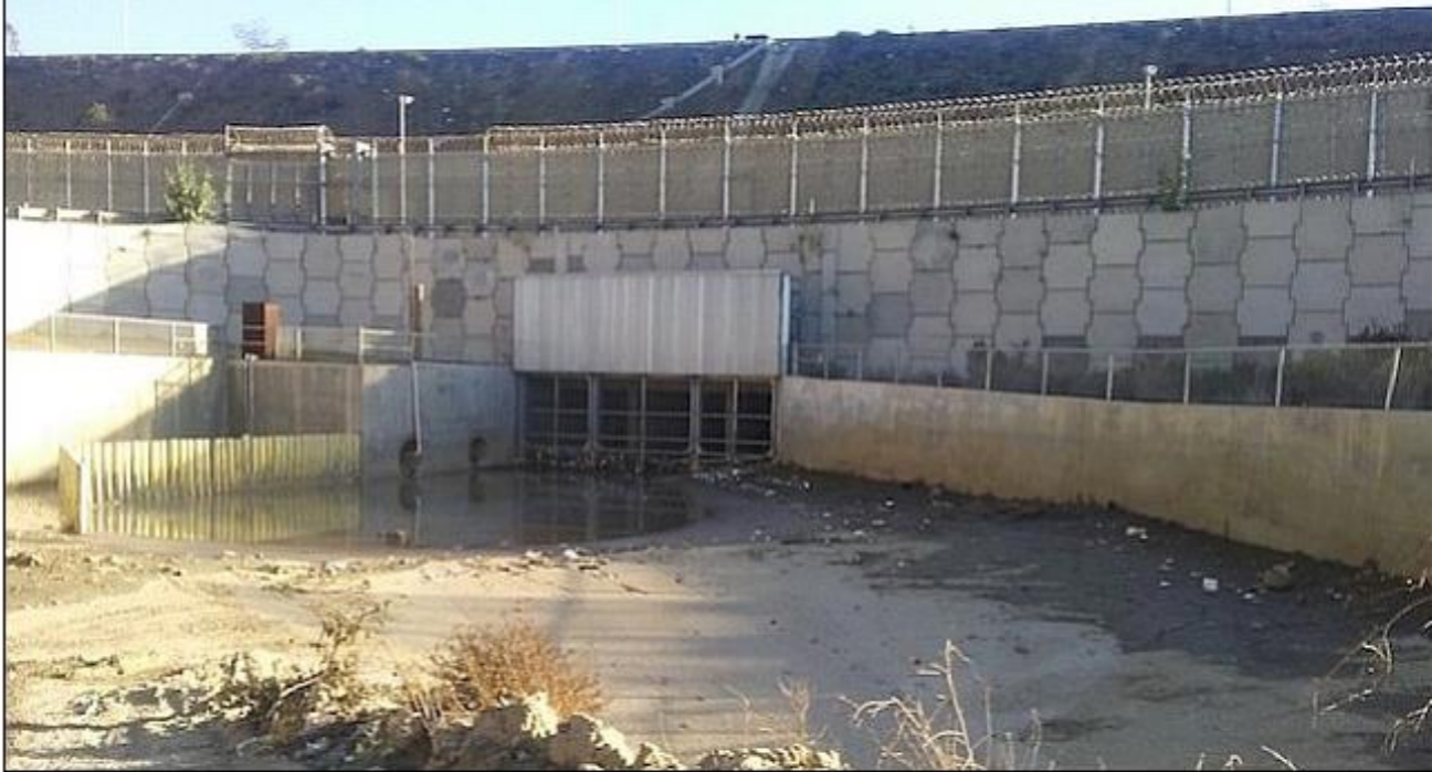
Goat Canyon culverts
